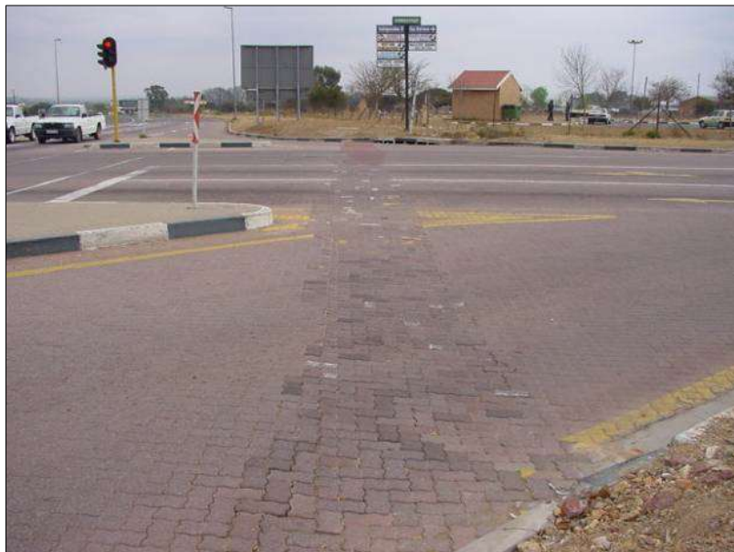
Figure D.4: Noticeable trench reinstatement on a block pavement
