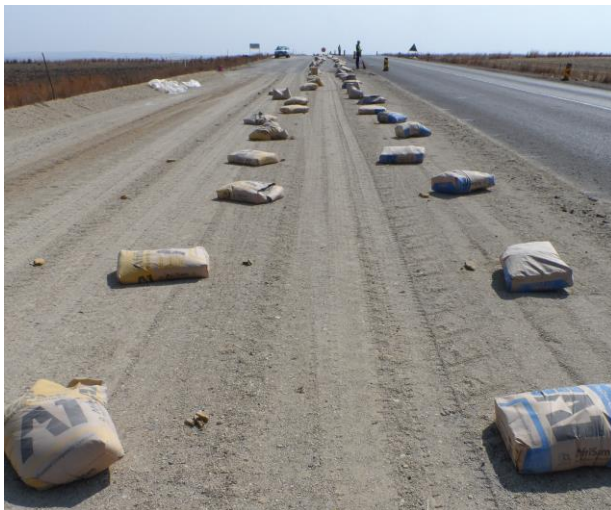
Figure 24: Two different types of cement being laid out for spreading
