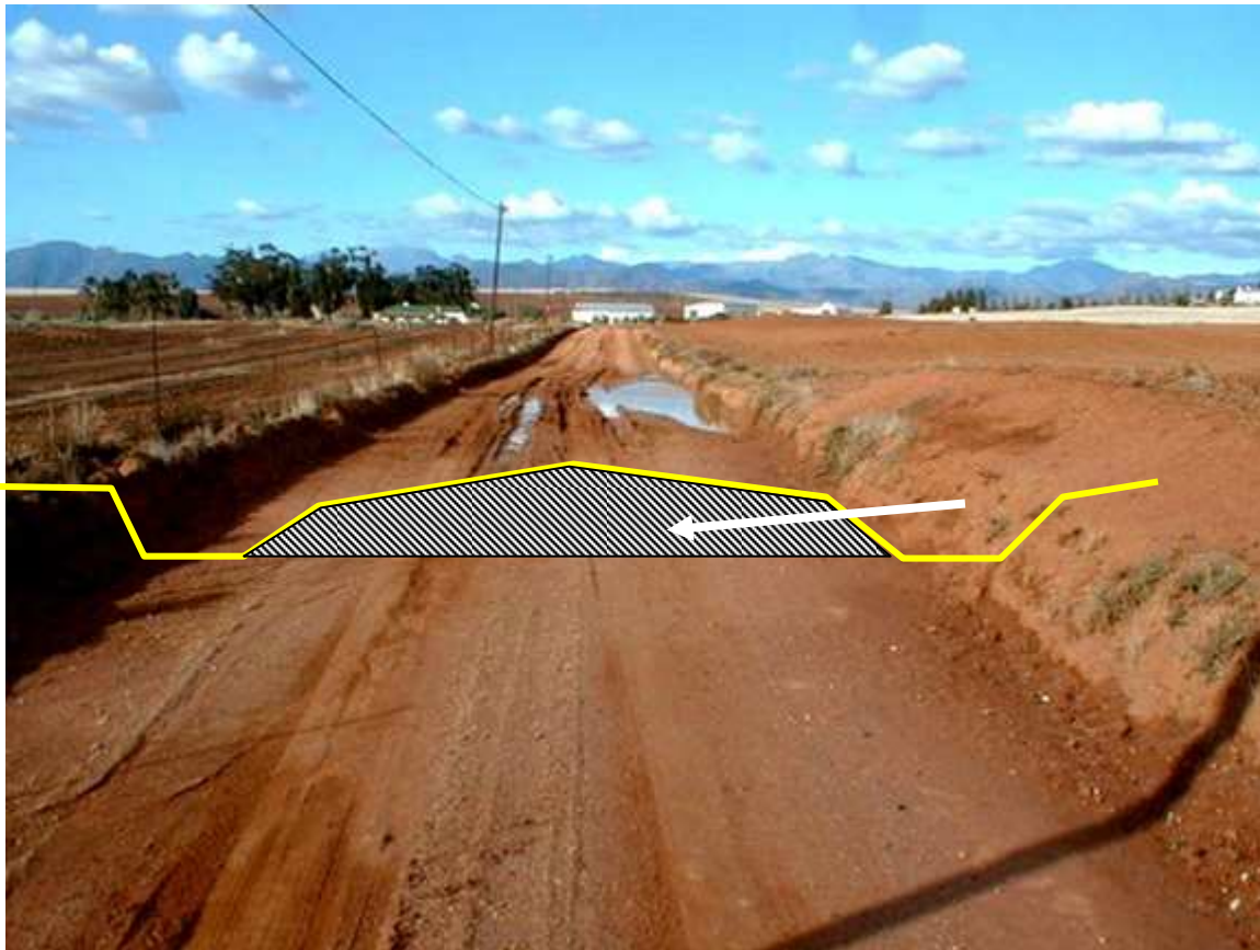
Figure 18 Forming to improve drainage
