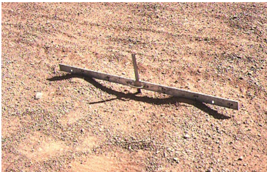
Figure 4 Typical example of loose corrugations
